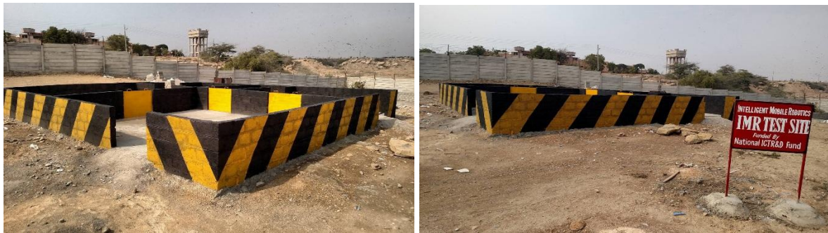
Figure 8.3: Fire Room at IMR Test Site
