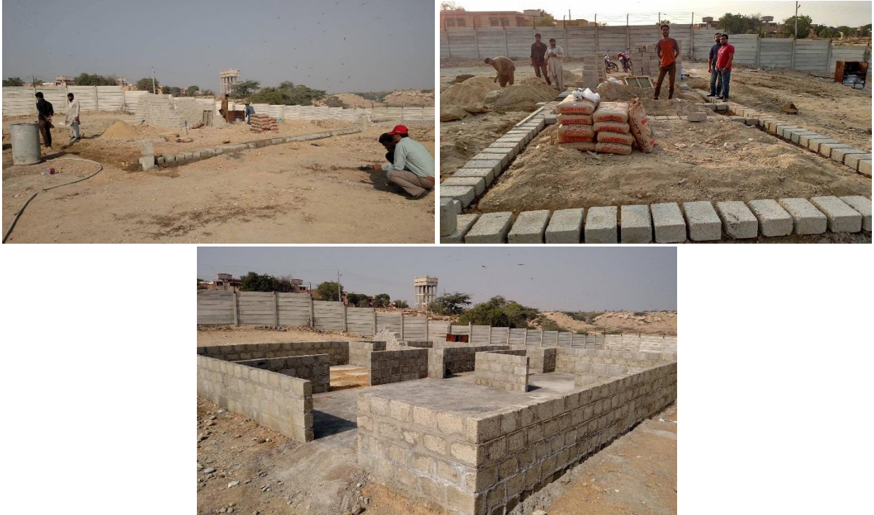
Figure 8.1: Setting Perimeter and Laying out foundation of the room
